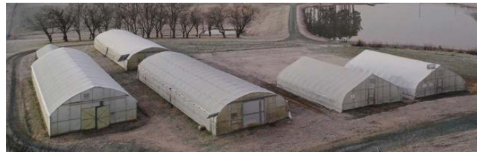
Figure 4-3. Single-bay high tunnels at the N.C. A&T State University Research Farm. From left to right: A Quonset and gothic hybrid fixed high tunnel (left), two Quonset fixed high tunnels (tandem) (center), and two gothic moveable high tunnels (side by side) (right).
