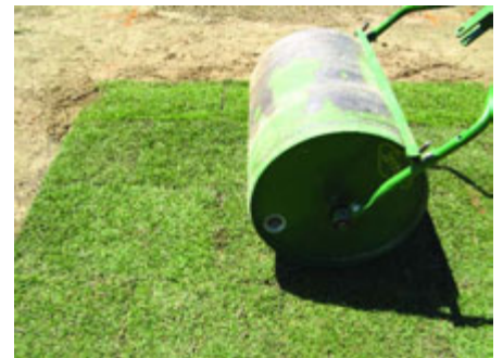
Figure 5. Rolling eliminates irregularities and establishes good contact between the sod and soil.
