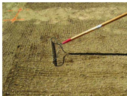
Figure 2. Loosening the soil to a depth of 0.5 inches prior to sod installation helps with rooting.
