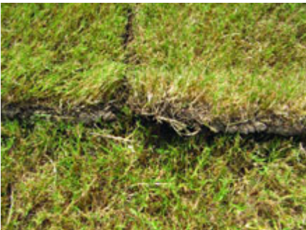
Figure 11. Overlapping sod seams during installation will cause desiccation.
