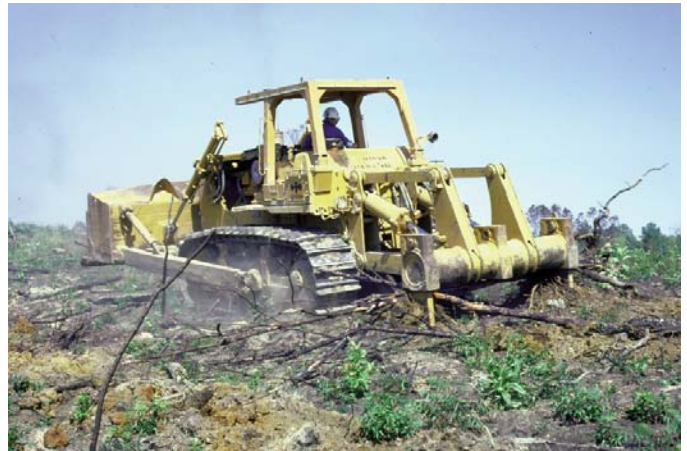
Figure 3. Ripping contracts must be carefully written to minimize the risk of site damage.
