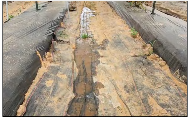
Image 3. Water flowing between rows, indicating a hole in the drip tape.
