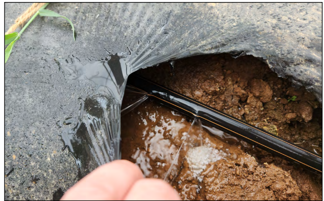
Image 4. Drip tape starting to split due to high pressure.
