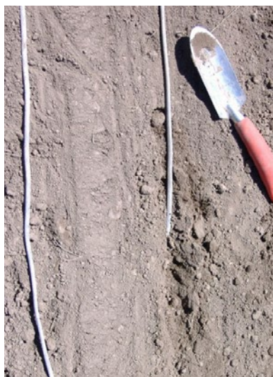
Image 4.31. Installing soil heating cables in a spinach bed inside a high tunnel.
