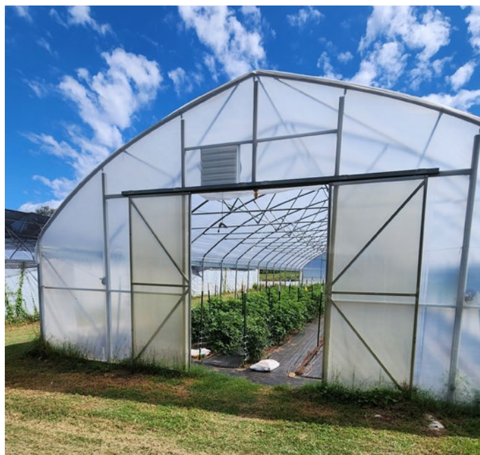
Image 4.23. An example of a popular endwall design in Arkansas. The wide door allows access for farm equipment, including small tractors, and promotes air flow into the tunnel.
