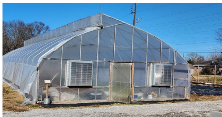
Image 4.28. A roof vent running the length of this tunnel.
