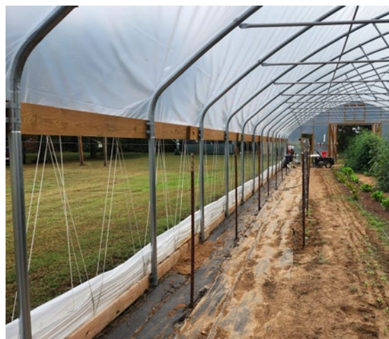
Image 4.20. Drop-down sidewalls on a gothic styled high tunnel.
