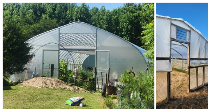
Image 4.27. Gable vents of different styles located near the peak on two gothic styled high tunnels.
