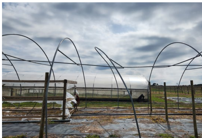
Image 4.24. Minor wind damage to a single hoop on a Quonset high tunnel.
