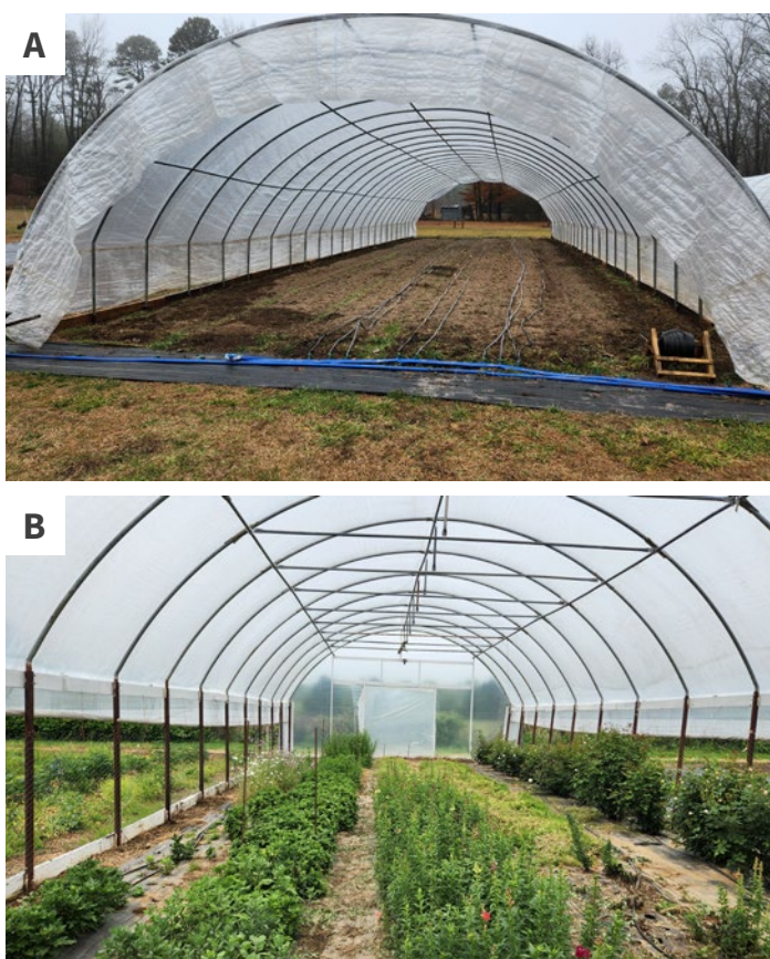
Image 4.4. Two Quonset styled high tunnels with extended ground posts. The sidewalls on the tunnel in Image A were extended 2 ft while the tunnel in Image B was extended 5 ft. This offers more protection for plants grown near the sidewalls in both tunnels as well as increases canopy space for taller crops.
