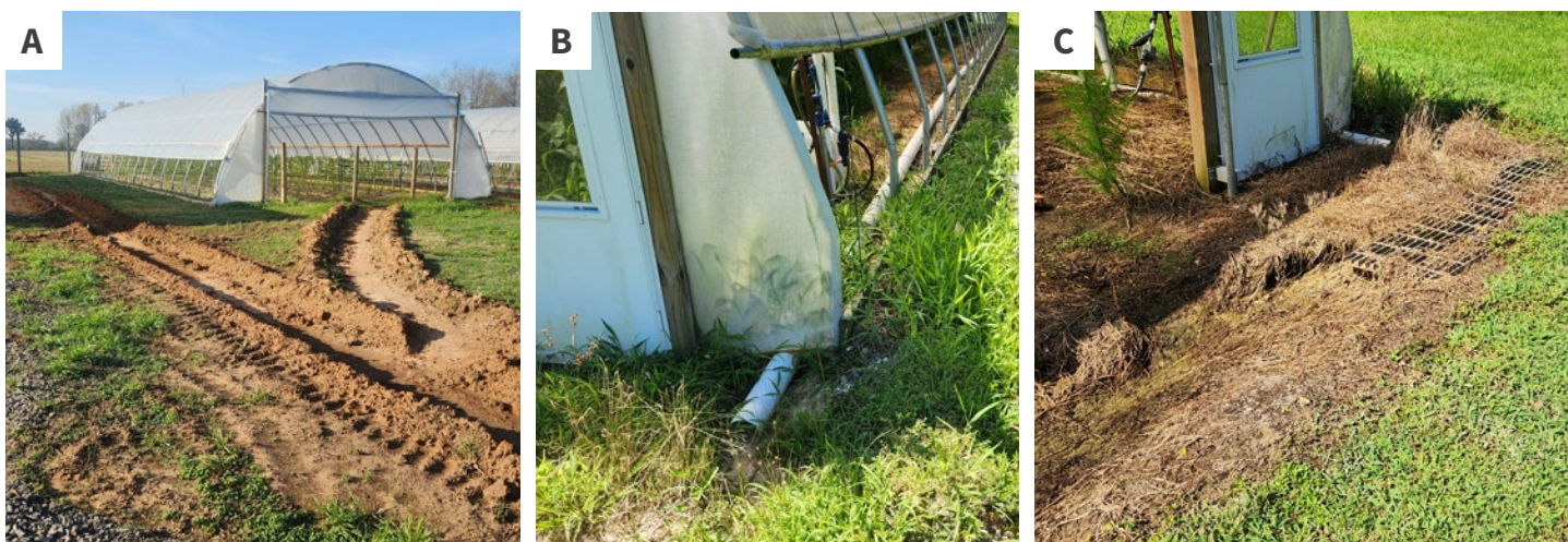
Image 3.7. Open drainage ditches to help divert water away from a group of high tunnels (A). A modified French drain installed inside a tunnel to help direct water out of the tunnel (B and C).
