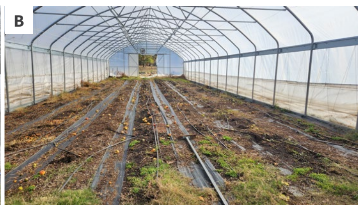
Image 2.1. A simple high tunnel design with minimal structural support (A). This simple high tunnel does have raised sidewalls which will be an added cost (A). A high tunnel design with additional structural support (trusses) and endwalls (B).
