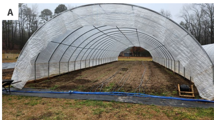
Image 2.1. A simple high tunnel design with minimal structural support (A). This simple high tunnel does have raised sidewalls which will be an added cost (A). A high tunnel design with additional structural support (trusses) and endwalls (B).
