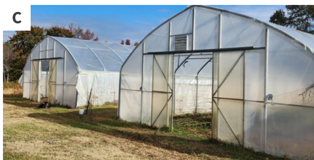
Image 4.22. Various endwall designs for high tunnels. Roll-up/down walls made with a woven plastic (A), hinged doors made with polycarbonate sheeting that swing open (B), sliding doors also made from polycarbonate sheeting (C) and a roll-up door with added structural support (D).
