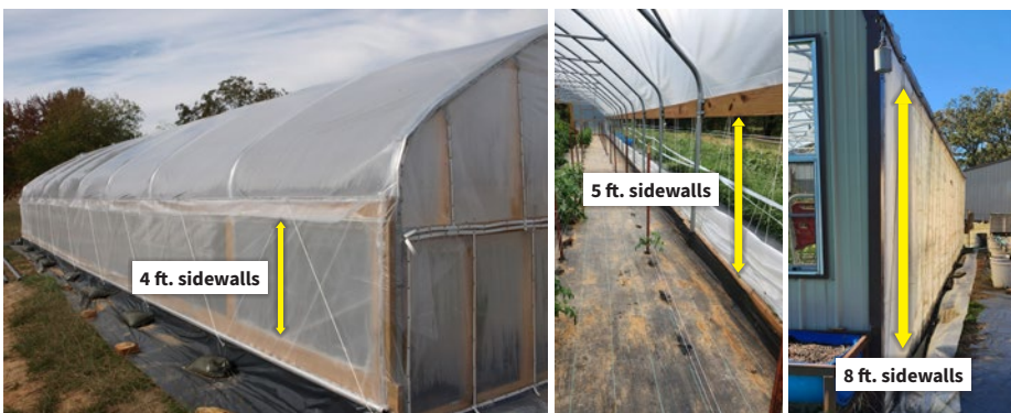
Image 4.18. Sidewalls with different heights. Sidewall height will have an impact on air flow inside the tunnel which will impact climate and disease management within the tunnel.
