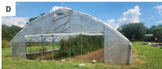
Image 4.22. Various endwall designs for high tunnels. Roll-up/down walls made with a woven plastic (A), hinged doors made with polycarbonate sheeting that swing open (B), sliding doors also made from polycarbonate sheeting (C) and a roll-up door with added structural support (D).
